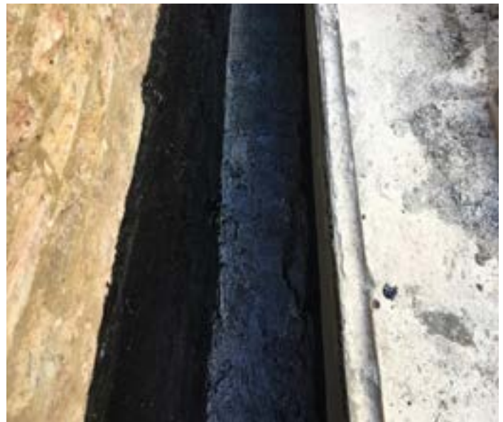
The external waterproofing also extended 1-metre below ground.
