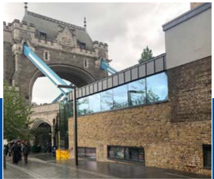
The Bridge Master's Quarters at No.1 Tower Bridge.
