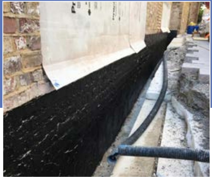
Newton 109-LM was extremely quick and easy to apply externally.
